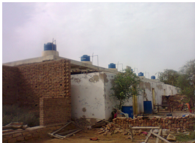
Water Facility Provided by Clariant at Chakhar Khan village
